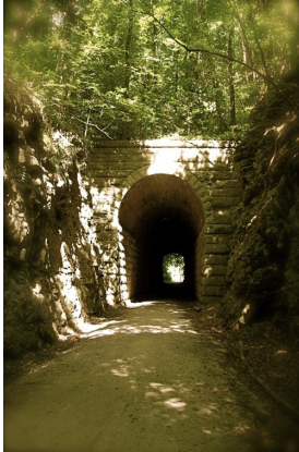
The Missouri, Kansas and Texas Tunnel in Rocheport
